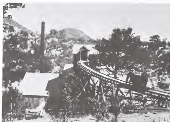
Figure 9. Ore was transported to the stamp mill by ore carts on rails. Photo courtesy Arizona Historical Society (AHS #72806).
